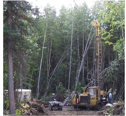
Drill Rig putting down a test well near the Cap’n Snow Center & Water Treatment Plant.
